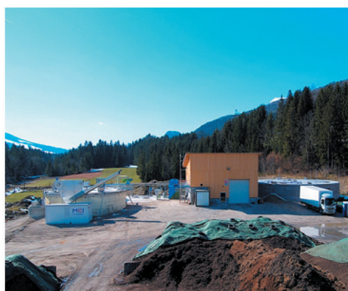
Figure 1, Biogas plant from "MUT" company in Kössen/Tyrol (Picture: "MUT" company)
