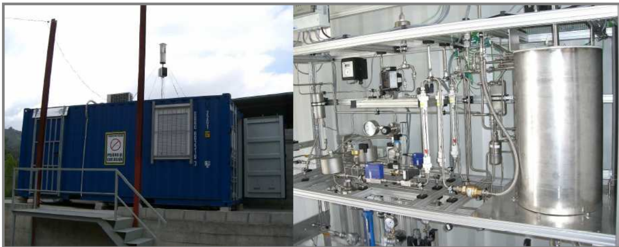
Fig. 1 Prototype for a biogas reformer at biogas plant in Frieres constructed by University Duisburg-Essen
