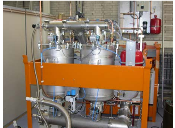
SOCOOL Trigeneration system under construction
